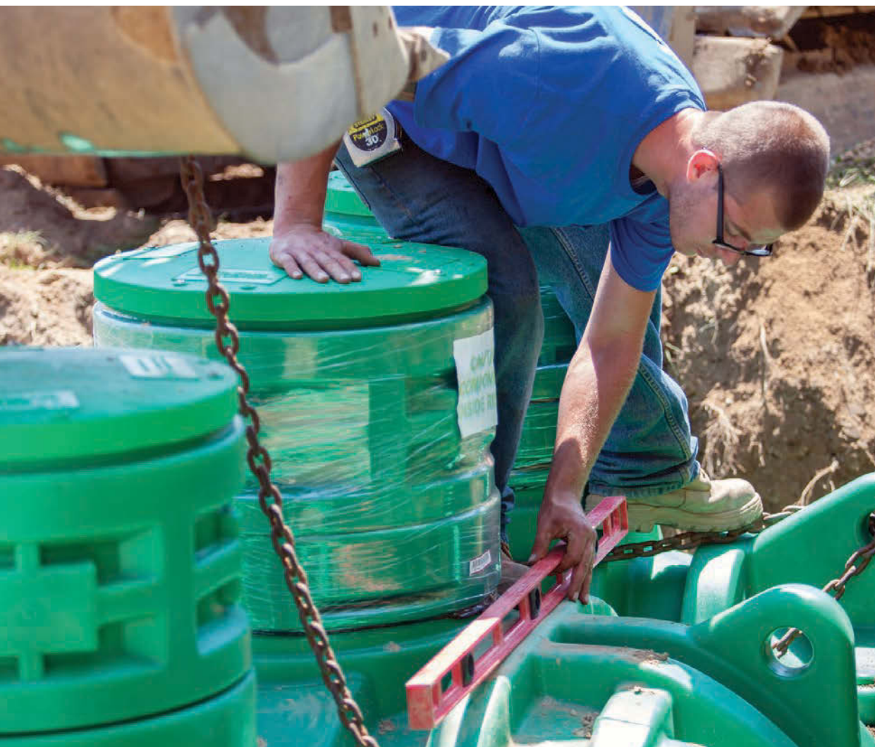
Dominic Cornwell checks the level of a Norweco Singulair Green unit after it was lowered into the ground.
