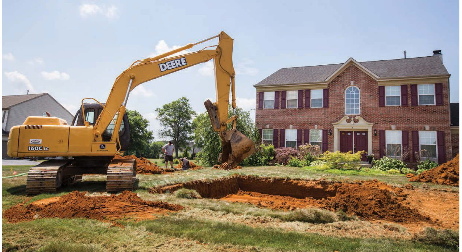
ABOVE: Gary Trull uses a John Deere 160C LC excavator to dig a drainfield for a replacement onsite system in New Jersey.
