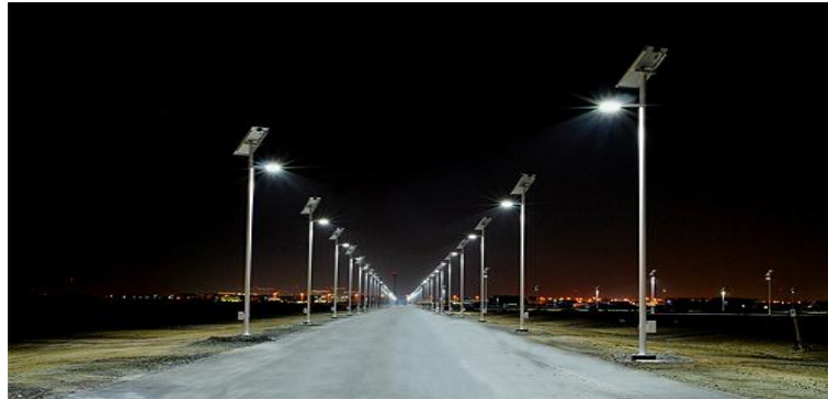
Fig :Shows every street lamps acting as a Li-Fi Hotspot.
